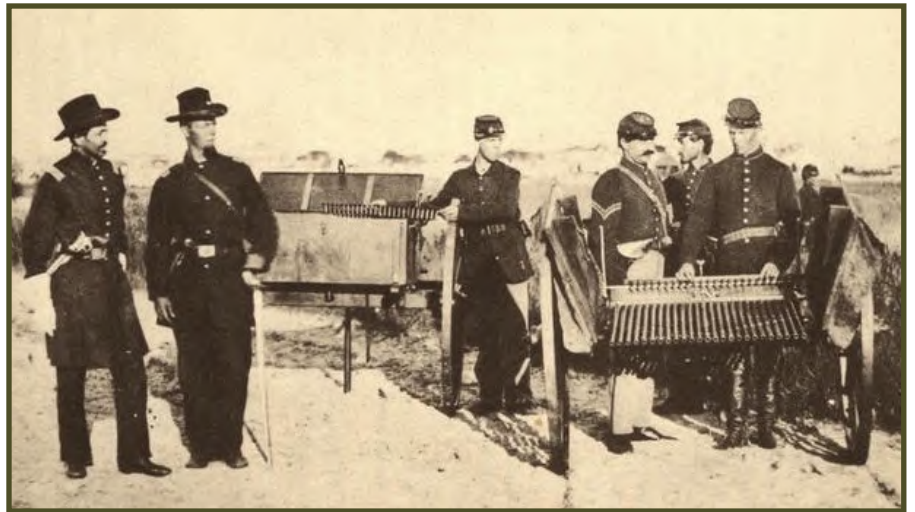
SECTION OF REQUA BATTERY THIRTY-NINTH ILLINOIS MORRIS ISLAND, SC 1863
